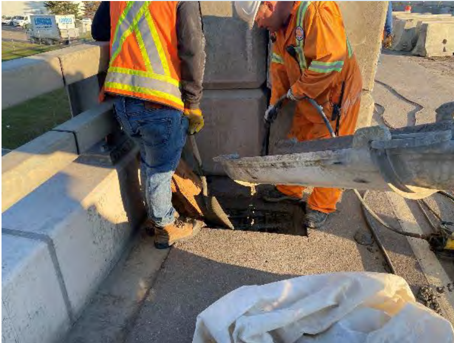
Pouring SCC Concrete Jacket
