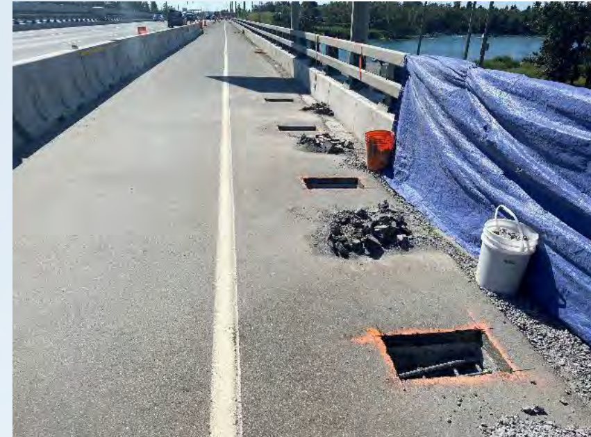
Deck Recession Cut for Pouring Concrete
