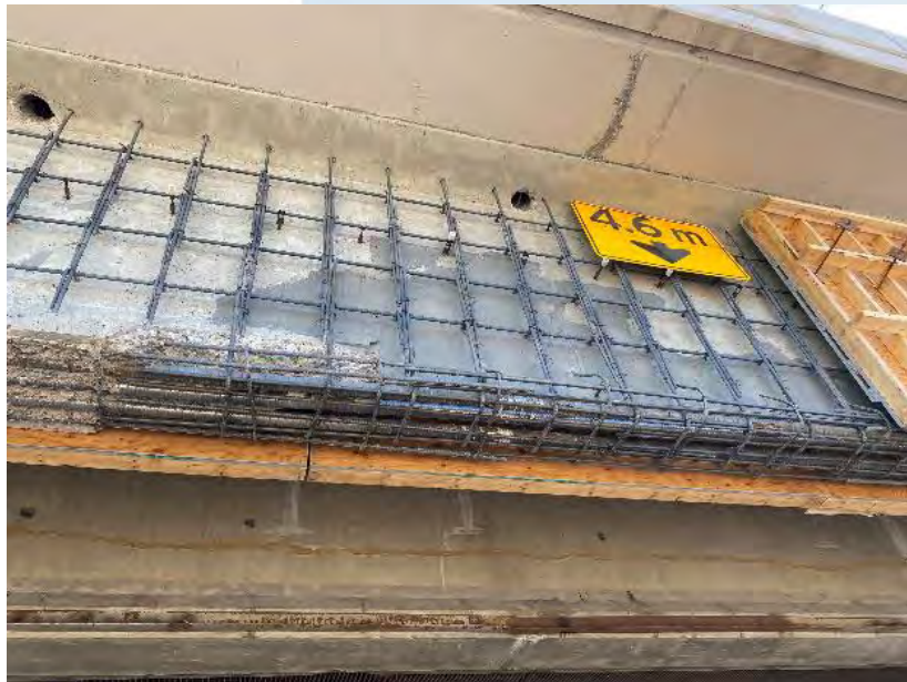
Reinforcing Steels/dowels for Concrete Jacket
