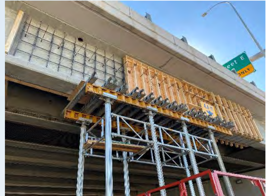
Formwork and Reinforcement for New Jacket
