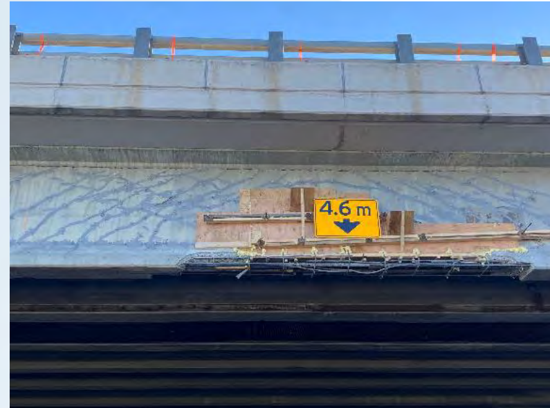
Formwork for Patch at Stage 1
